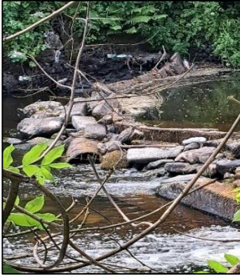
(iv). Barrel dam
