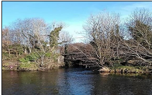
1 The Viaduct & Lugton Mou'
