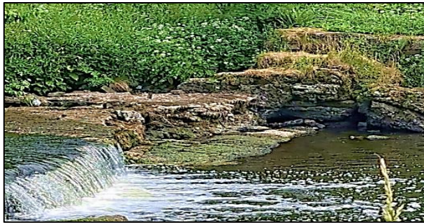
(vi) Jeanie's dam & Mill Lade masonry
